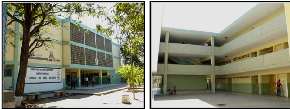
Figure 8. Box-Type school building inspected in Sucre State
