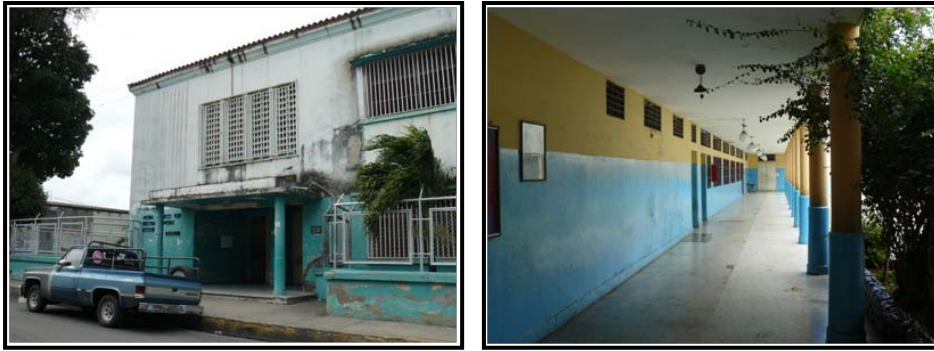
Figure 6. Old school building inspected in Sucre State
